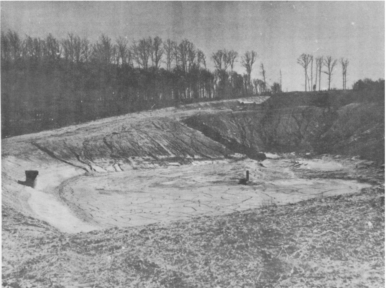
Figure 7-1. Sediment basin on a construction site.
